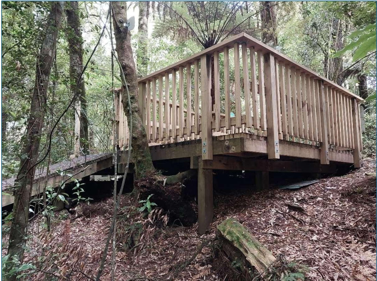
Figure 1 Example of zip line launch platform
